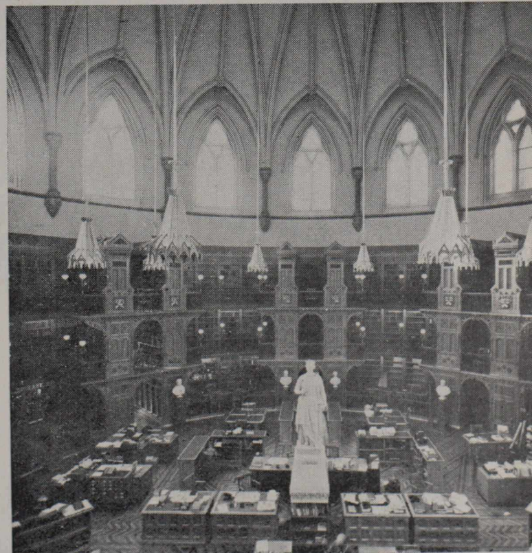
The vaulted Hall of Honour (upper right) leads from Confederation Hall to the door (background) of the Parliamentary Library. Right, the Parliamentary Library.
