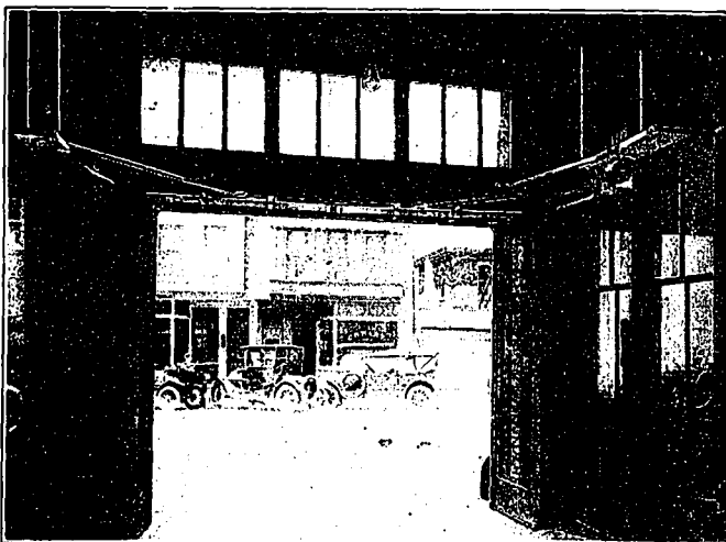
ELECTRICALLY OPERATED GARAGE DOOR.
