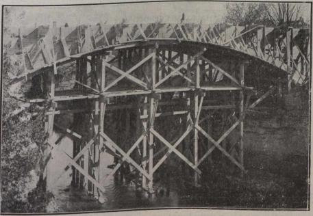
Fig. 1 .- Showing Superstructure of Bridge.
