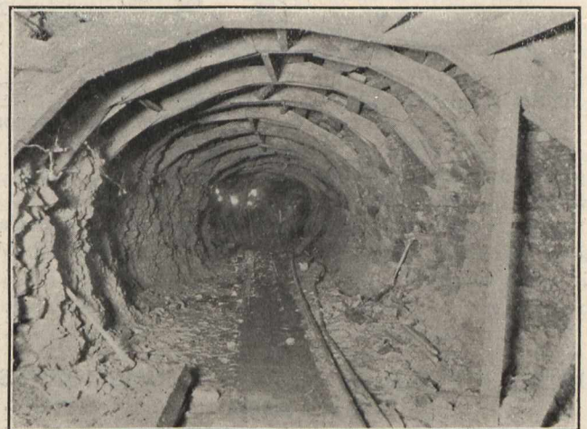
Tunnel Showing Timbering.
