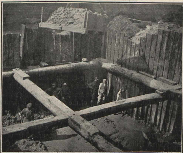
Sheet Piling, Shaft No. 1.
