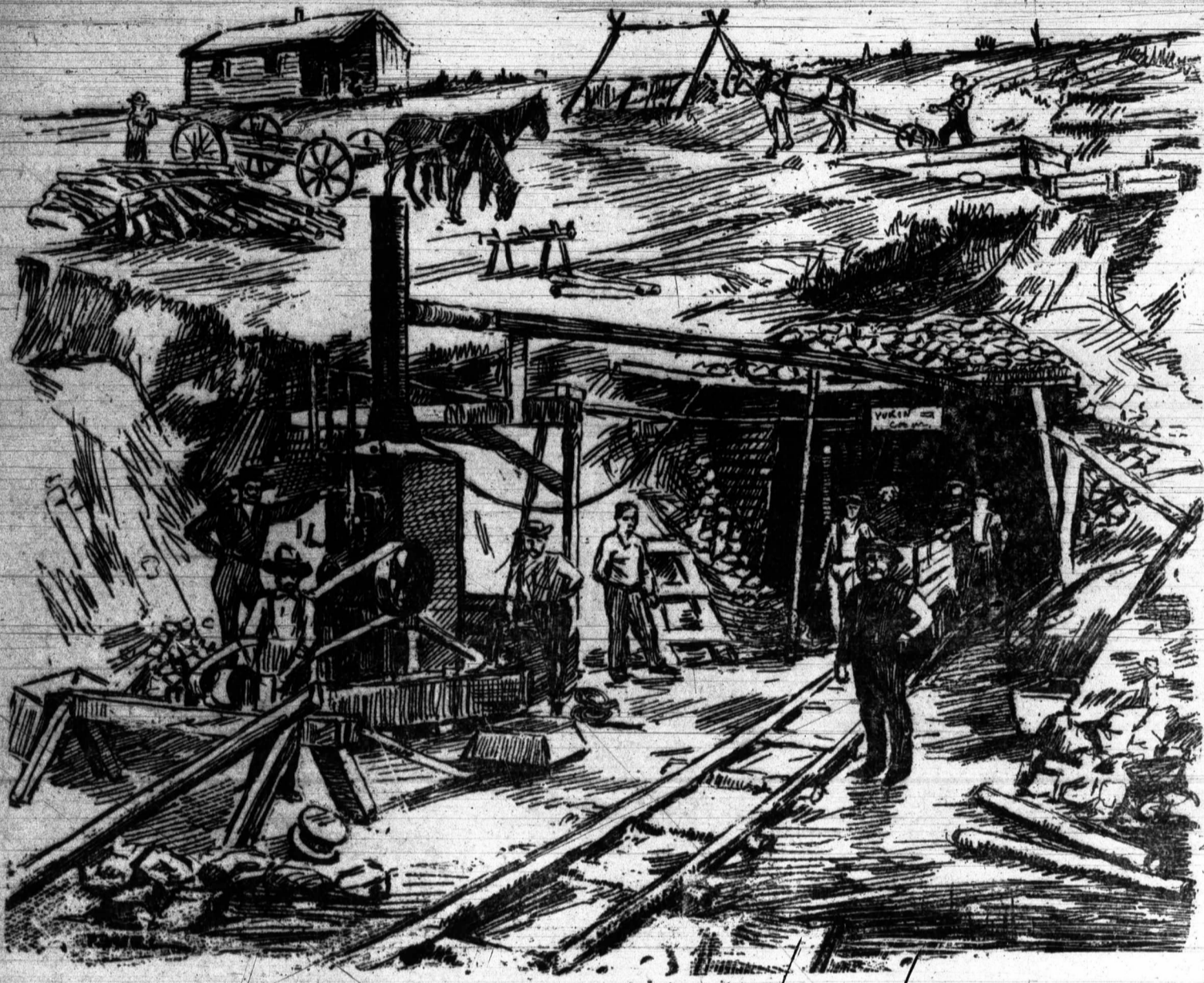
View of tunnel No. 1 on the property of the Yukon Gold Fields, Limited; R. B. Wood, manager.
