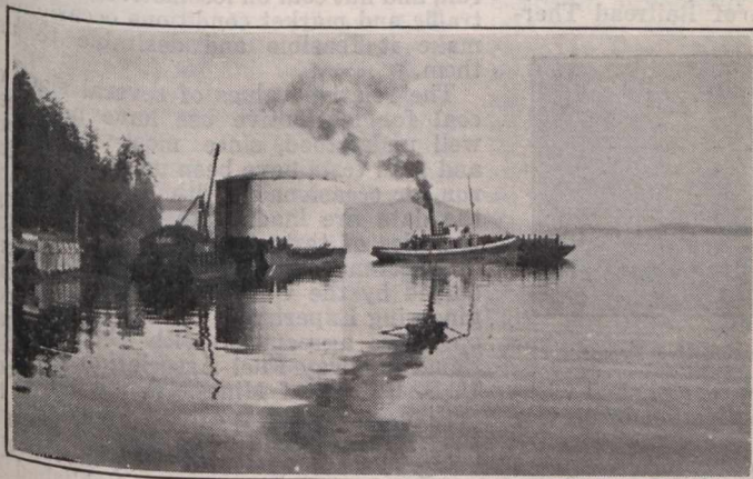
Moving Oil Tanks in British Columbia.
