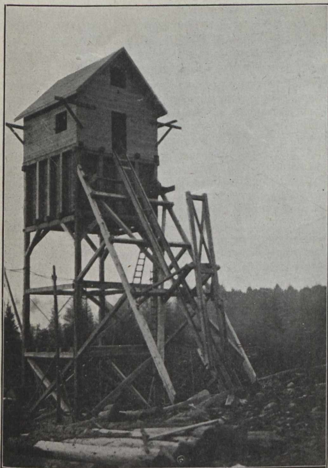
Head frame at Tough-Oakes Mine, Kirkland Lake, Ont.
