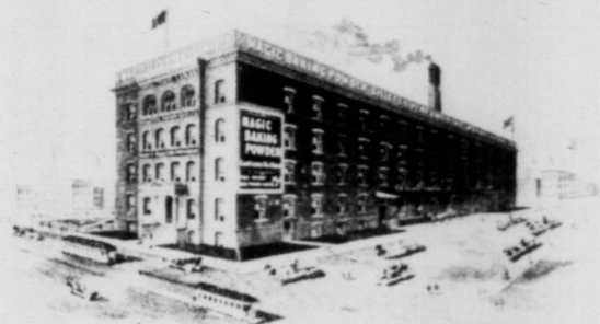
GILLETT BUILDING KING, DUNCAN AND PEARL STS TORONTO, ONT.
