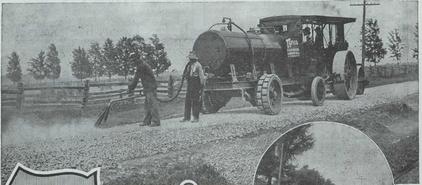
Applying "Tarvia X" on Kennedy Road, Scarborough Township, Ont. Toronto and York Roads Commission. The view in the circle is the finished road. Note smooth, dustless surface.
