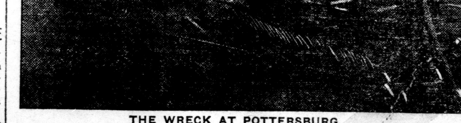
THE WRECK AT POTTERSBURG. When the express struck the freight, the caboose of the latter was knocked into kindling-wood, and thrown to one side. The smokestack, sand-chest, cowcatcher, etc., were ripped off the locomotive. At the other side of the telephone poles can be seen a freight car, where it was thrown on its side, the trucks standing on the ground alongside the tracks.
