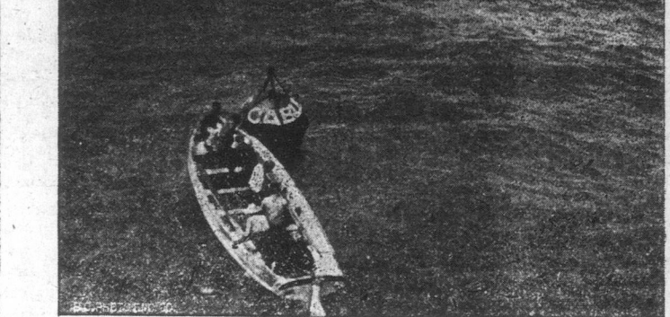
BUOYING THE CABLE.
