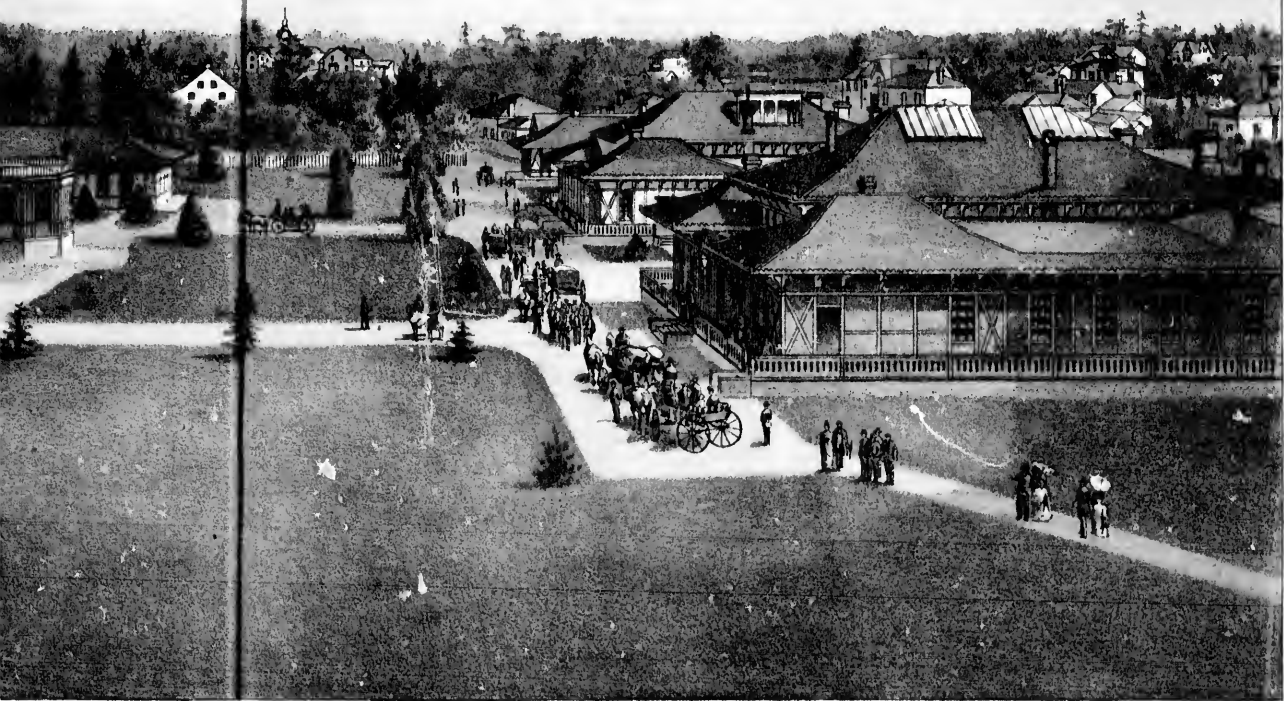
• THE GOVERNMENT BUILDINGS VICTORIA B.C. •
