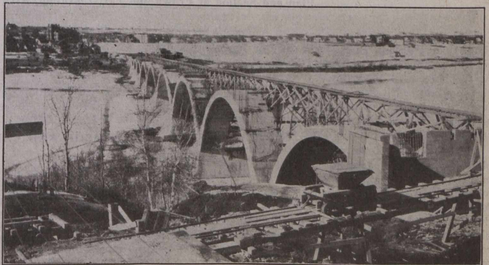
East Abutment. Centering Removed. Before Pouring Spandrel Columns or Floor System.
