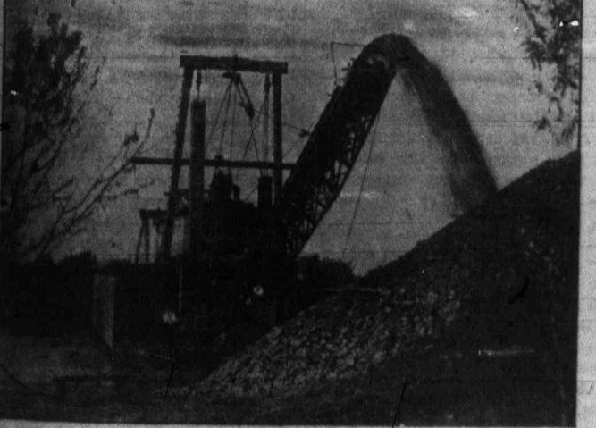
Steam Dredge Operating in Connection With a Conveyor.
