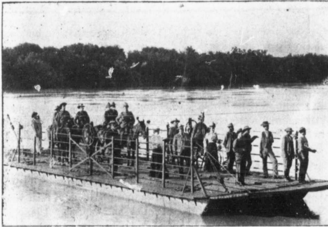
FLOATING BRIDGE ACROSS SOUTH AFRICAN RIVER.
