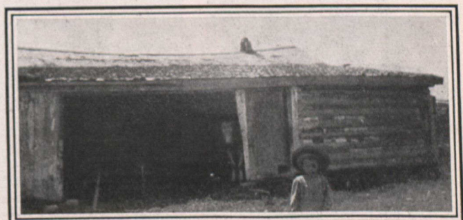
First Mission House in the Ing Parish.
