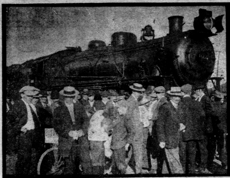
Photo by Hines. Grand Trunk Freight Locomotive No. 562, Which Left the Rails at Clarence street crossing Saturday afternoon, burying her wheels almost axle deep.
