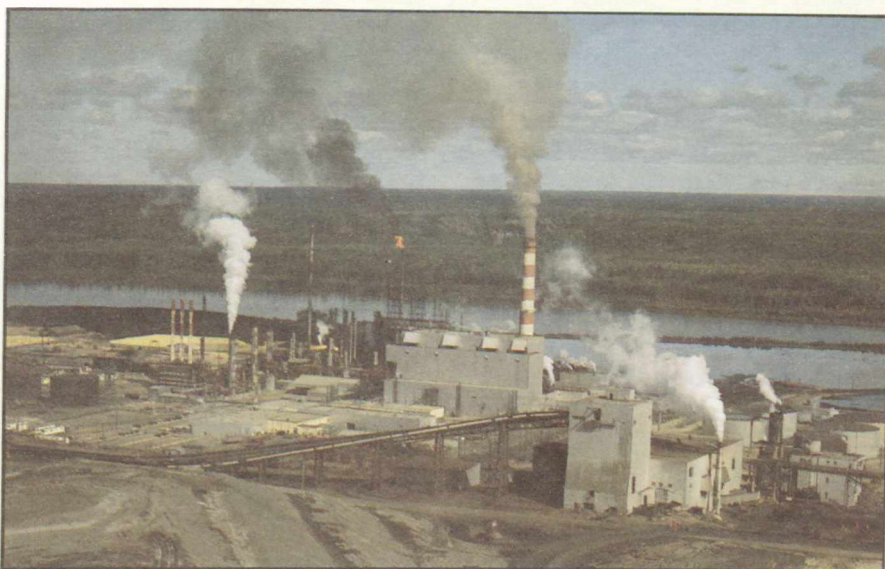
The Suncor synthetic oil plant at Fort McMurray is the largest point source of sulphur dioxide emissions in the province of Alberta, releasing 93,000 tonnes annually.
