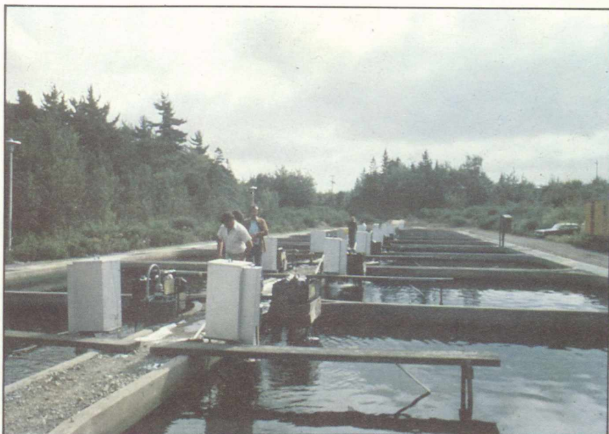
This salmon hatchery in the Mersey River, Nova Scotia had been completely destroyed by high water acidification levels. The introduction of limestone chips in cribs has restored it to a successful operation.
