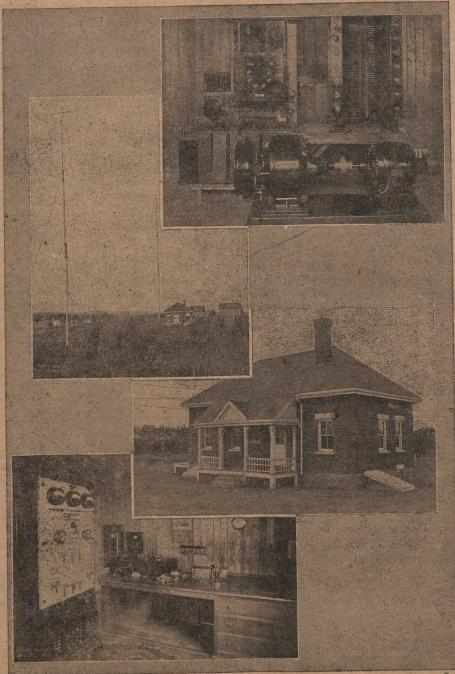
Complete Transmitting Apparatus at an up-to-date Radiotelegraph Station Canadian Government Station, Port Arthur
