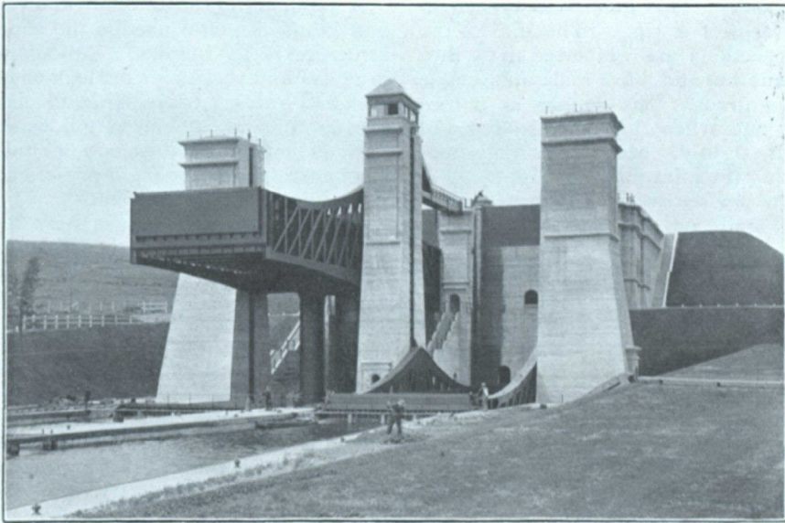
THE PETERBOROUGH LIFT LOCK—FROM THE LOWER REACH
