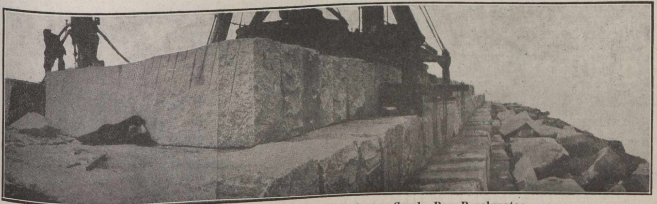
Fig. 1.—Drilling Holes for 30-ton Capstones, Sandy Bay Breakwater.
