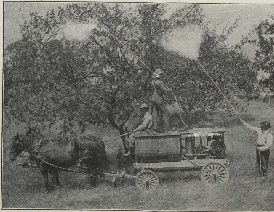
A Power Spraying Outfit suitable for use in Large Orchards and on Tall Trees
