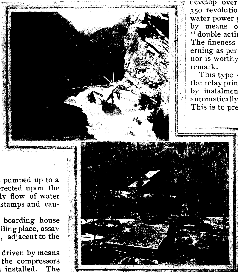
1. THE DAM AND FLUME. 2. MILL AND OTHER BUILDINGS.
