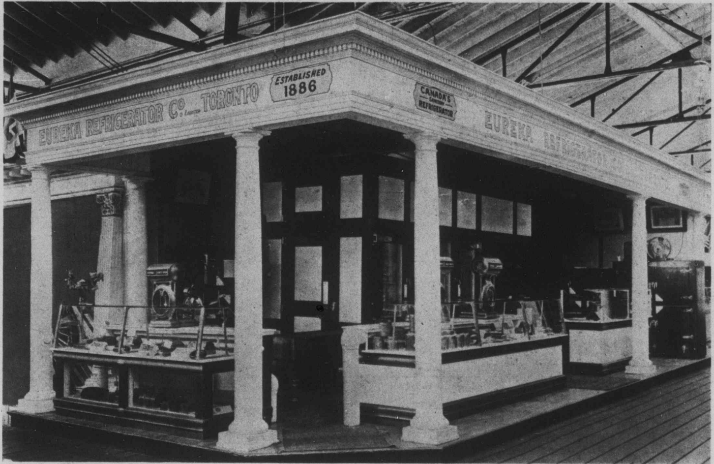
The Suggestive Equipment Exhibit of the Eureka Refrigerator Co.
