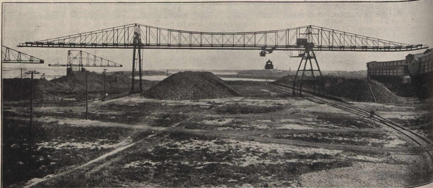
ASTORIA LIGHT, HEAT & POWER CO., ASTORIA, N.Y. SHOWING BRIDGE TRAMWAY.
