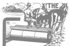
Has a strong, rigid frame with three drums. It is fitted with a heavy steel axle and roller bearings. The drums, made of heavy, steel plate, are riveted up to stand any strain. The frame is stiffened with double truss rods. It pulls and turns easy, and there is no neck weight.
