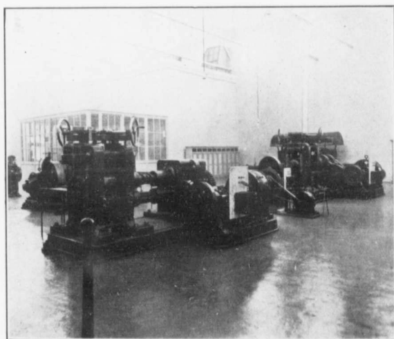
Fig. 10—Rolling mills. Fillet-annealing furnace on right.
