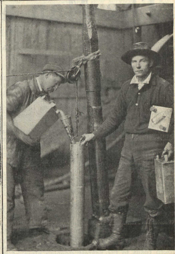
Charging an Oil Well With Nitro-glycerine. Familiarity breeds contempt in the handling of this dangerous explosive.
