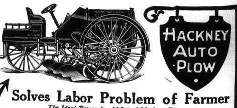
The Ideal Power for 160 to 640 Acre Farms The only "One Man Machine" on the market that can be used for plowing, as a stationary engine for power purposes, and as a tractor for hauling loads, etc.
