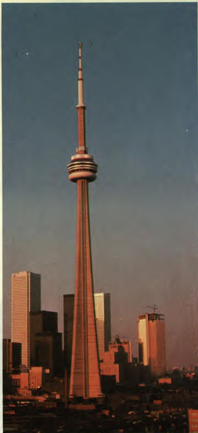
The CN (Canadian National) telecommunications tower in Toronto, at 1,800 feet, is the tallest free-standing structure in the world. It has broadcast facilities for television (UHF, VHF and cable), FM radio and microwave transmission.
