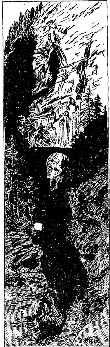
FIRST BRIDGE ON THE VIA MALA.
