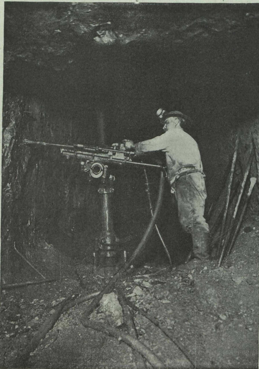
Operating a Leyner Drill with old style bit in, the Calumet and Hecla Mine
