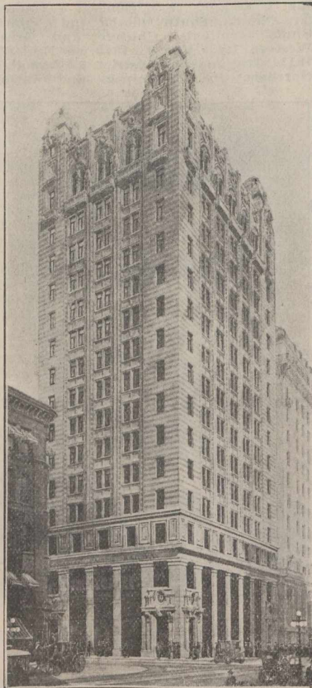
Canadian Pacific Railway Office Building, King and Yonge Streets, Toronto.
