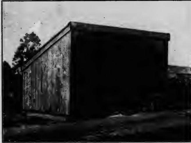
Another poor poultry house. The windows are too low, causing the floor to be cold and draughty during the winter months.
