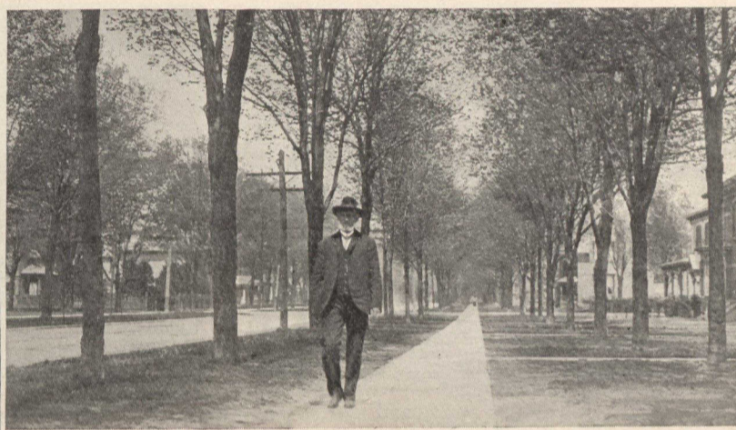
Vansittart Avenue, Woodstock. Evidences of "the town beautiful" may here be seen in the laying of cement walks, removal of fences, grading of lawns and boulevards, and the planting of trees.
