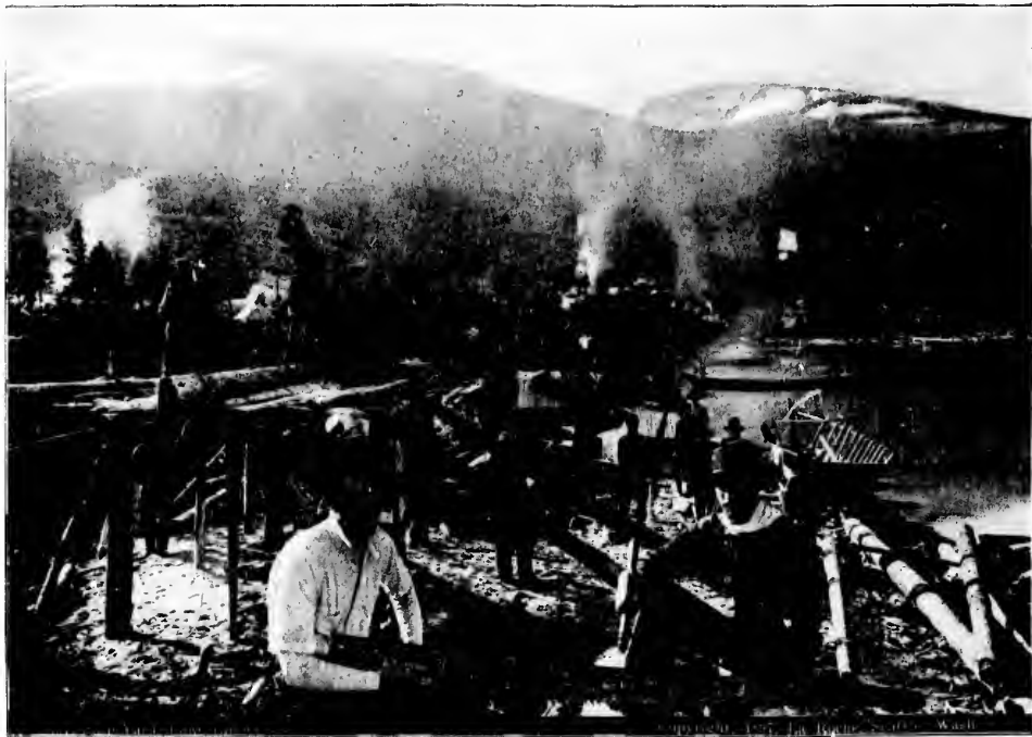
SHIP YARD, LAKE LINDERMAN.—Without a doubt this was the busiest scene along the whole route. Scores of men were here, always at work constructing boats for descending the waterways to the Yukon. Timber is found in the immediate neighborhood and logs of about seven inches in diameter are cut to the necessary lengths, rolled upon a staging and whipsawed into the required shape. Thus a week or more is employed in building a boat for the long journey north. Assuming that they are handy with tools, four men can take the standing spruce, saw out lumber and build a boat large enough, in a week, to carry them and 4,000 pounds of provisions; and it should be a good staunch boat at that.
