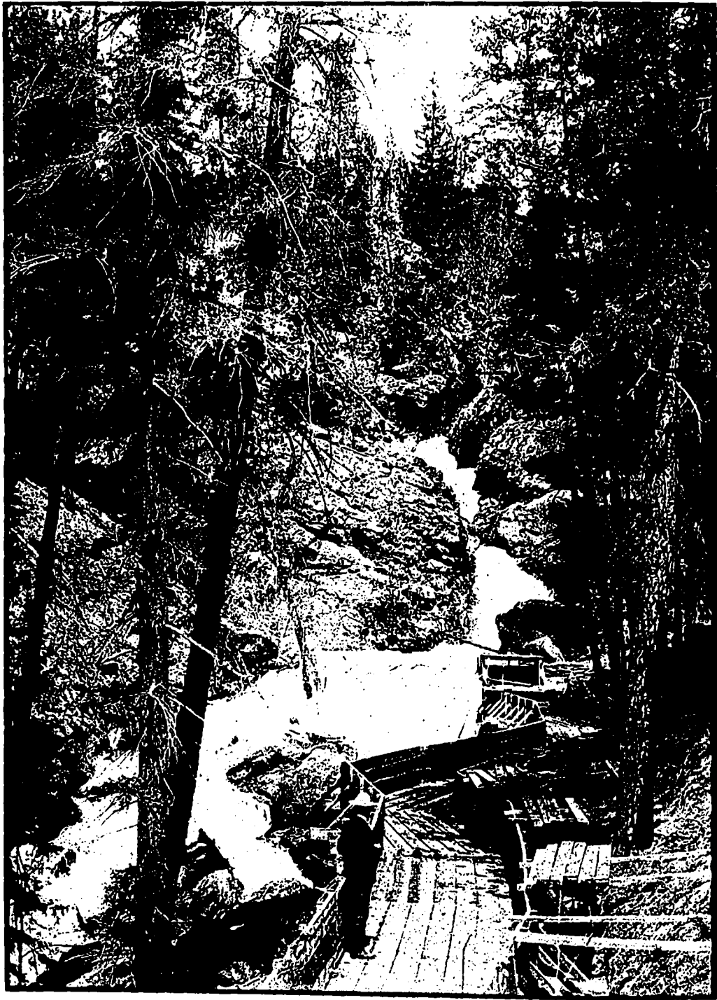
Head Gate Central Okanagan Coy's Irrigation System.
