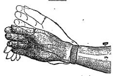
The above cut represents an Artificial arm with Ball and Socket Wrist Joint, recently invented and manufactured by Geo. R. Fuller, successor to the late Dr. Bly, of Rochester, N. Y.
