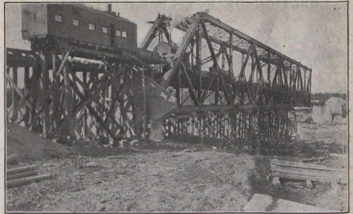
South Flanking Arm in Place; Cantilever Erection
