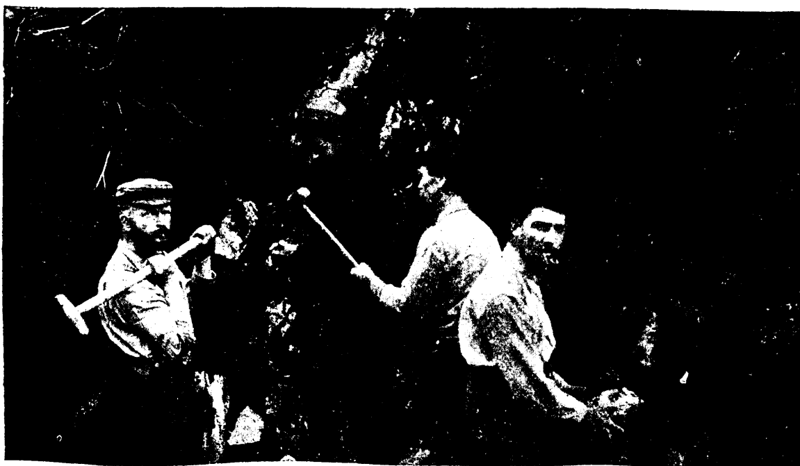
COMMENCEMENT OF TUNNEL, 7-FOOT LEDGE, GOLDEN EAGLE, ALBERNI.
