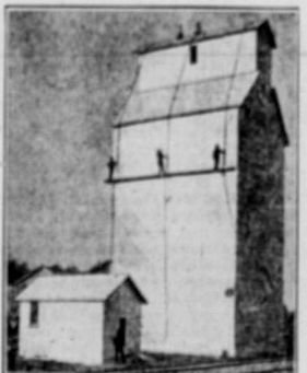
The Standard Elevator built by the Gillespie Elevator Construction Company.
