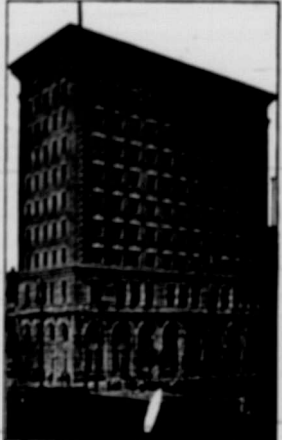
Union Bank Building, Winnipeg
