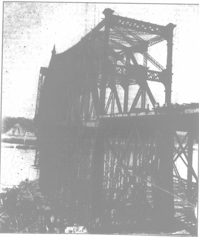
No. 1.—The Quebec Bridge, Showing the "Falsework" or Scaffolding; and Upper Braces of 20 thicknesses of Steel.
