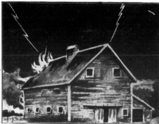
UNPROTECTED—Ruined in a Moment.
