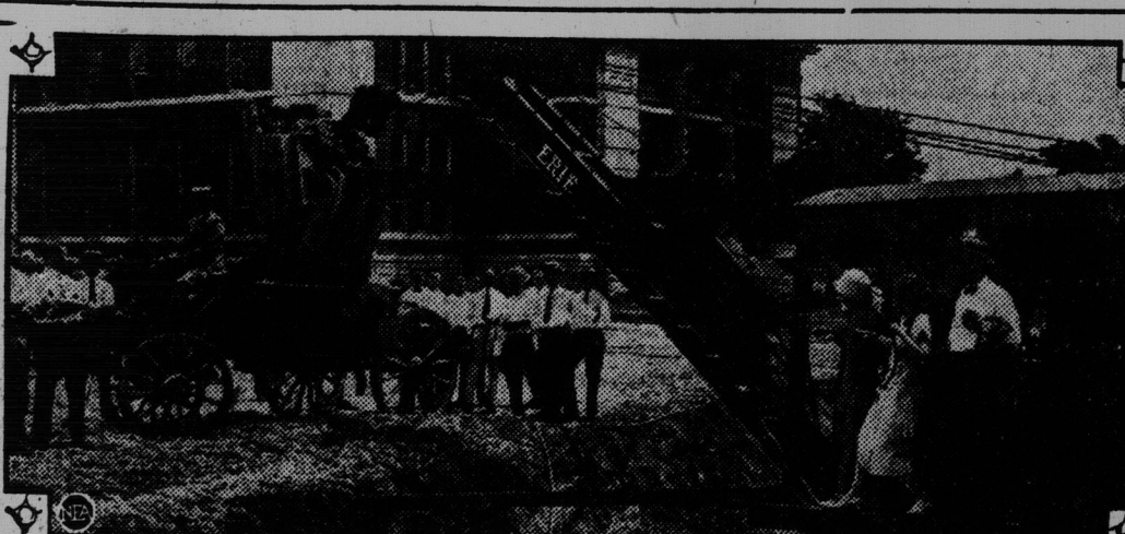
This shows ground being broken for the first of the new buildings of the Duke University at Durham, N. C. Duke University, formerly Trinity College, has been endowed with $600,000 by J. B. Duke, wealthy tobacco king. Photo shows Sibyl Flowers, daughter of Prof. R. L. Flowers, pulling the cable that released the first shovelful of dirt. Prof. Flowers is driving the dirt wagon. Dr. Frank C. Brown, who holds the chair of English in the university, is standing behind Miss Flowers.
