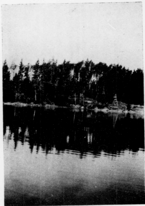
Taken by W. J. Ireland. WINNIPEG RIVER—WHITEDOG FALLS—CABLE STATION— SOUTH CHANNEL.
