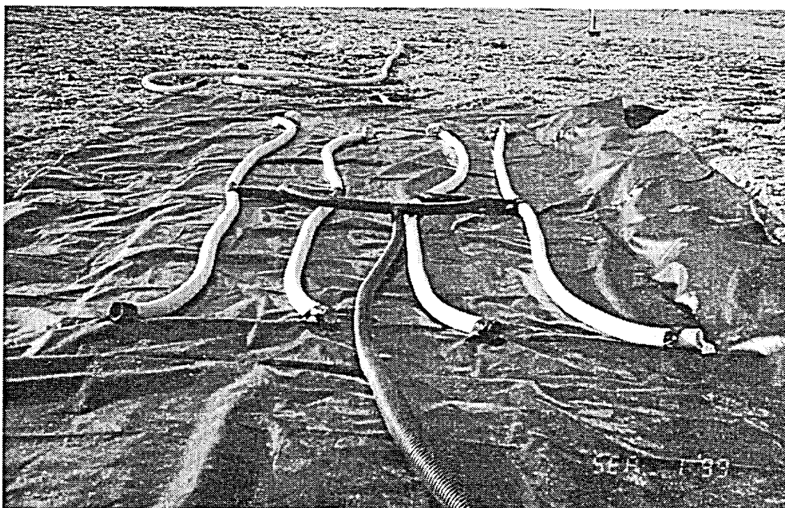
Figure 3. Placement of vapour extraction/aeration system piping on HDPE liner prior to bio-cell berm construction.
