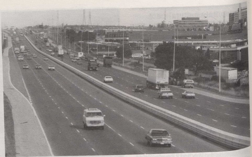
IBC highway barrier snakes along Highway 400 north of Toronto.
