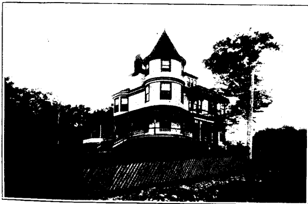
Residence of Miss E. Scarfe, Dartmouth, N.S. NEPONSET Papers used in this building. Architects, Harris & Horton, Halifax, N.S.
