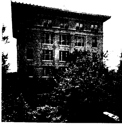
Civil Service Building, Washington, D.C. "ALCA" Lime replaced white cement for brick mortar. Interior plastered with "ALCA" Lime
