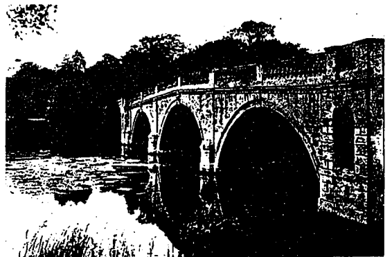
Bridge, Renaissance Type, in Cumberland Park, the Dukeries.
