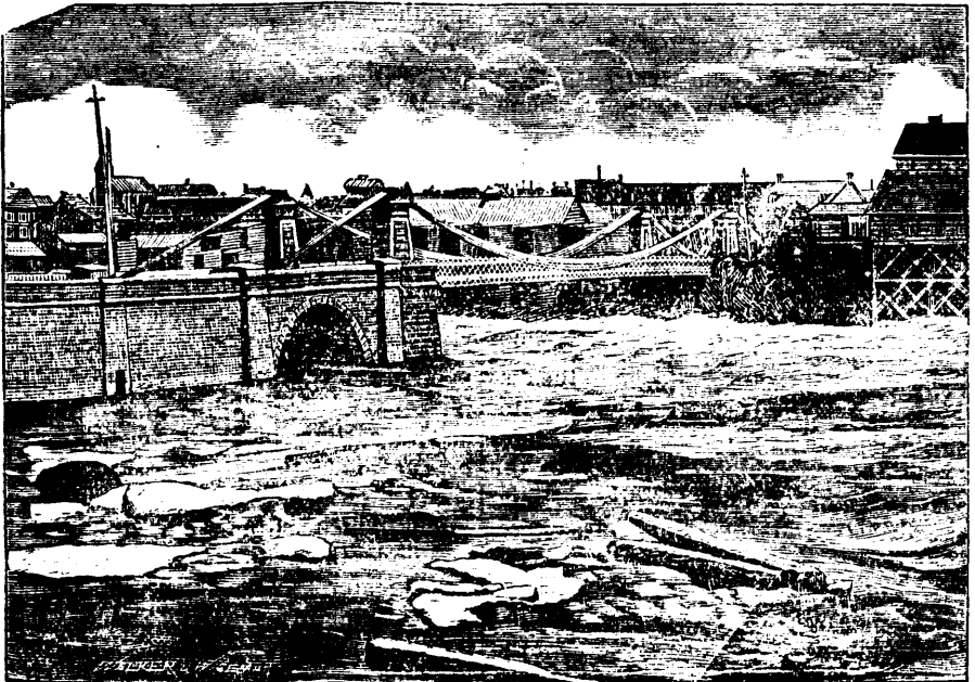
SUSPENSION BRIDGE, SAW MILLS, ETC.
