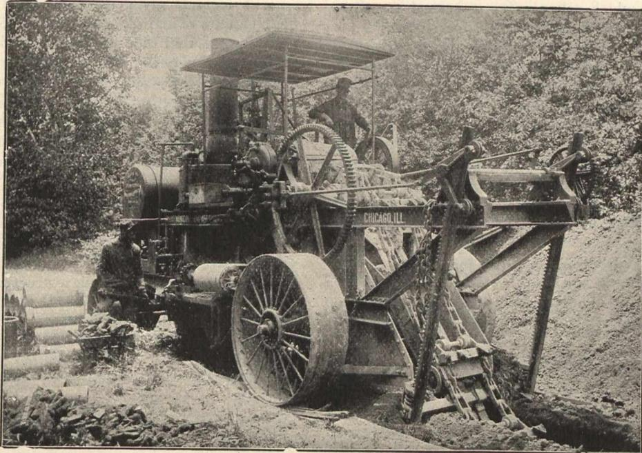
abled to introduce to our readers a modern trench machine of the wheel type, which is undoubtedly one of the most economical digging appliances ever invented. They are made in five sizes, excavating trenches any depth to twenty
