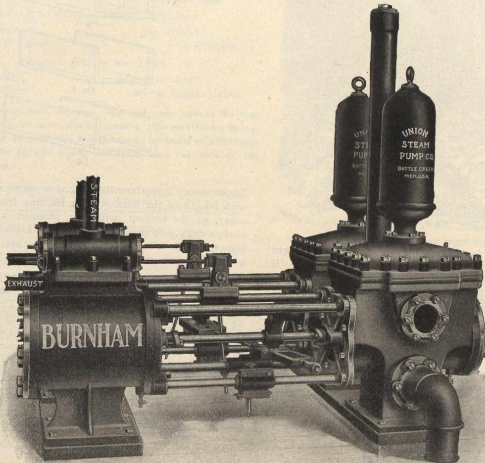
will give some idea of their advantages. The pumps are single cylinder, double acting, and are so arranged that they will operate together, or independently. The valve motions on both pumps are connected by a centering bar, and so arranged that when one pump is at the end of the stroke,
