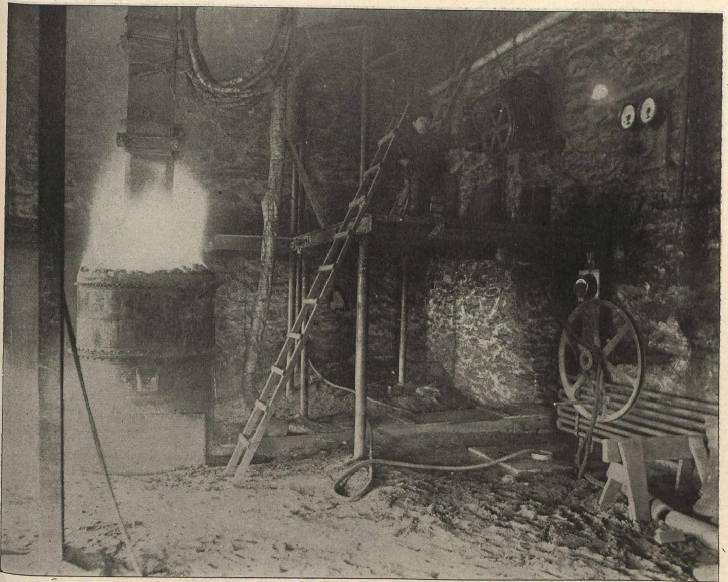
Electric Furnace, showing Method of Regulating Electrode and Measuring Instruments in Place.
