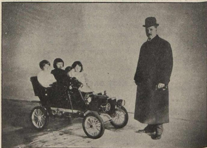
has two speeds forward, and one reverse, power being transmitted to the rear axle by a Cardan-shaft. The tonneau is detachable, has two side-doors, and accommodates four passengers as shown in the picture. All levers and pedals necessary for a perfect control are provided, also two brakes and five lamps. As will be noted, a baby-chauffeur has been trained to run the automobile, which is the smallest working model ever produced, weighing only 243 pounds.
