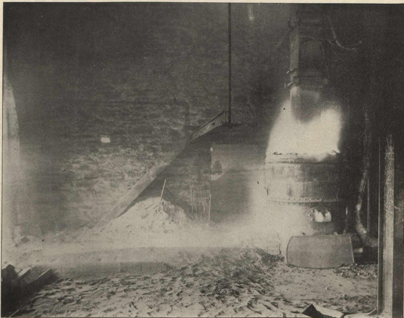
Showing Electric Furnace just after Metal has been Tapped.
